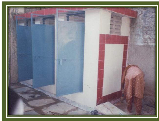
Toilets Constructed by Municipal Corporation through Leaders' Initiatives
