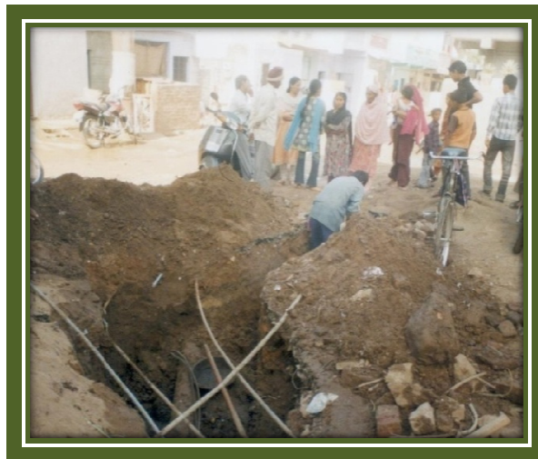
Drainage Work undertaken by Municipal Corporation through Community Pressure
